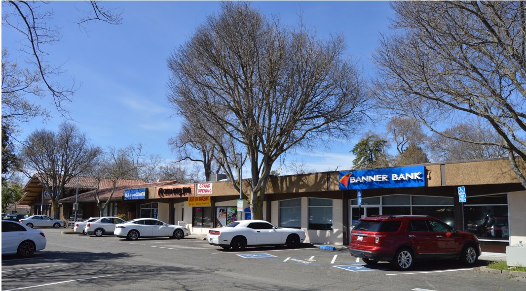
Figure 1. Storefronts facing parking lot at south elevation of 335 F Street, looking northwest.
